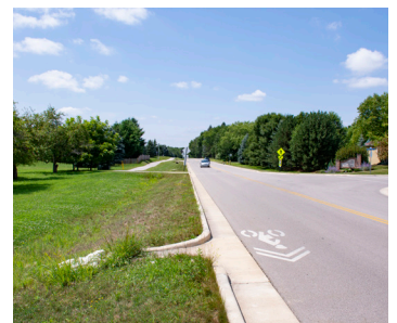
Allen Road Grass Swale System
