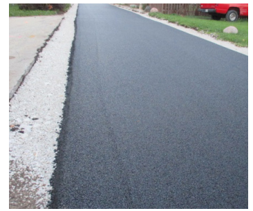
Buena Park Alleyway Porous Pavement
