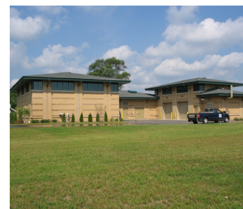
Well 10 Iron and Manganese Filtration
